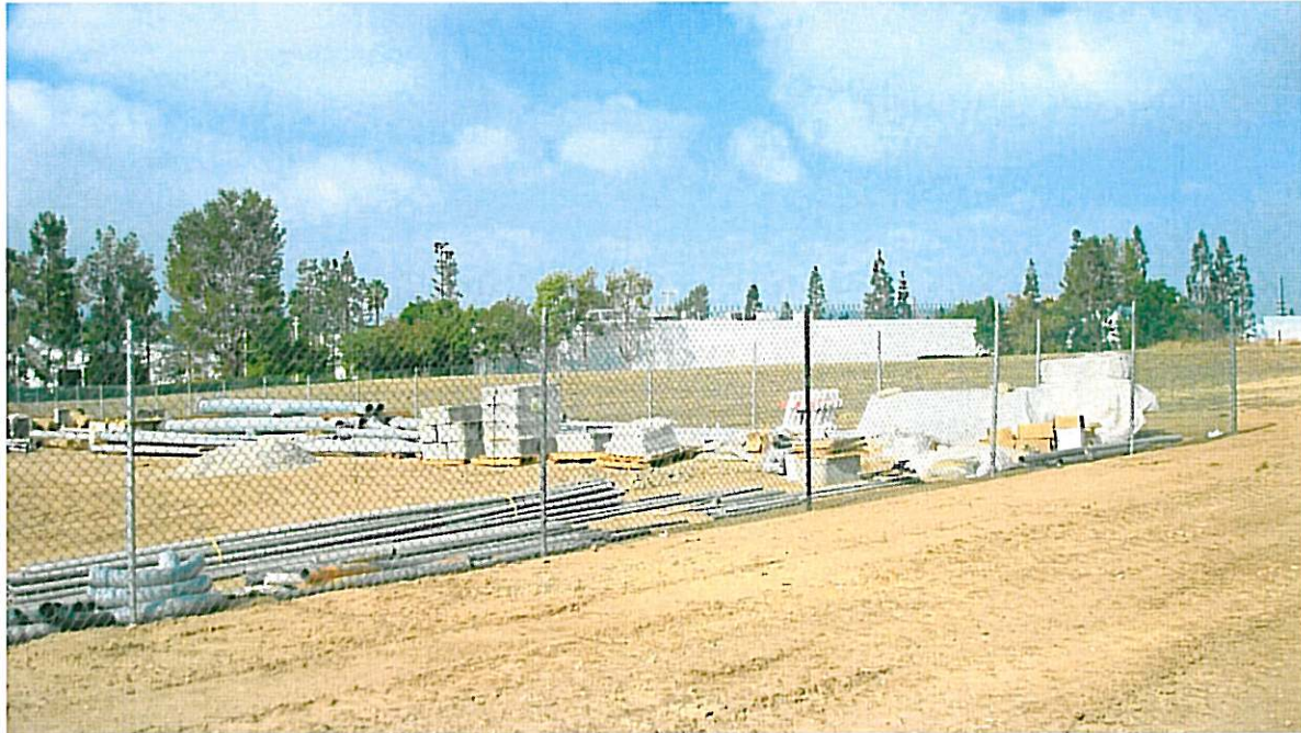
Property facing northwest
