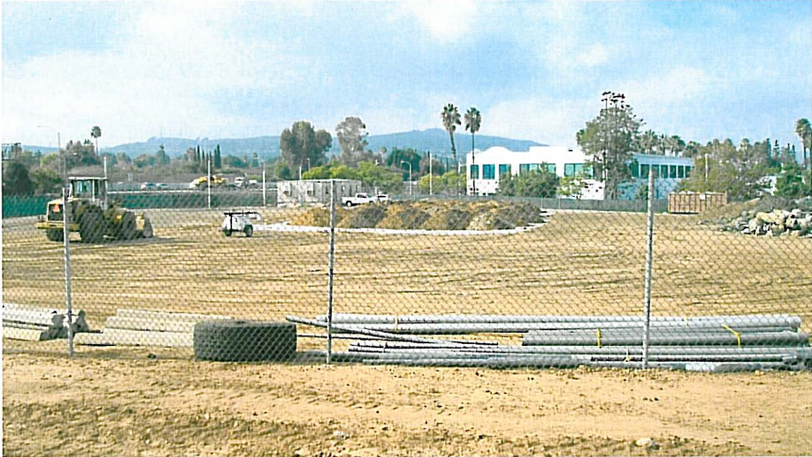
Property facing southwest
