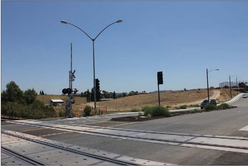
Photograph 1: Looking southeast into Project Site at new Charlie Road detour railroad crossing at north end of Project Site
