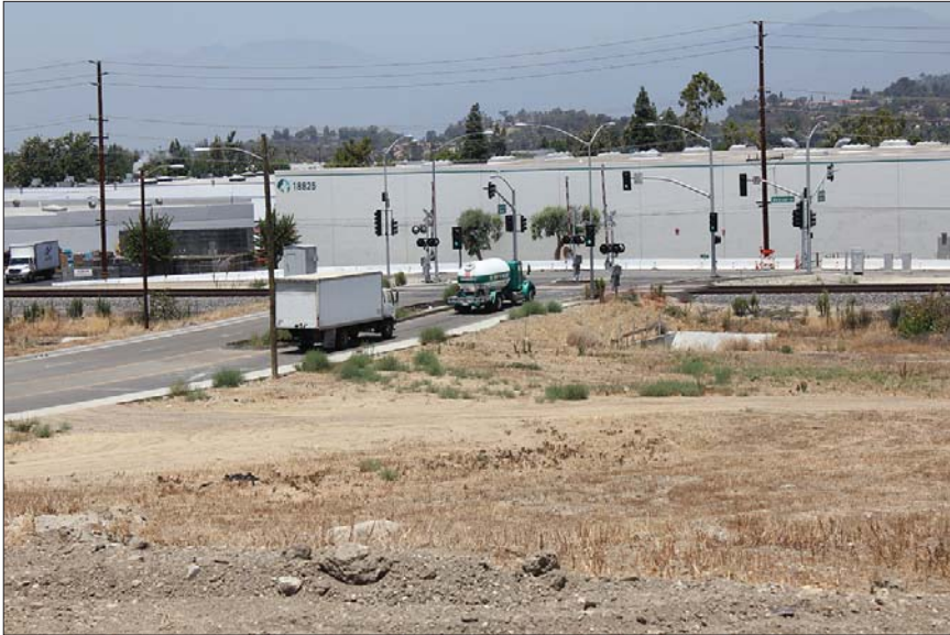
Photograph 1: Looking north at Charlie Road detour railroad crossing and storm drain culvert at Railroad Avenue, north end of Project Site
