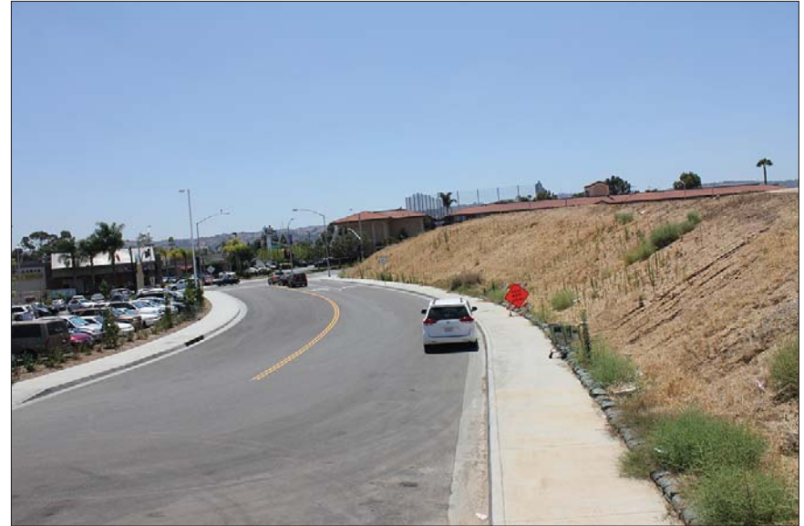
Photograph 2: East edge of Project Site along shared driveway 99 Ranch Market Shopping Center (looking south toward Gale Avenue)
