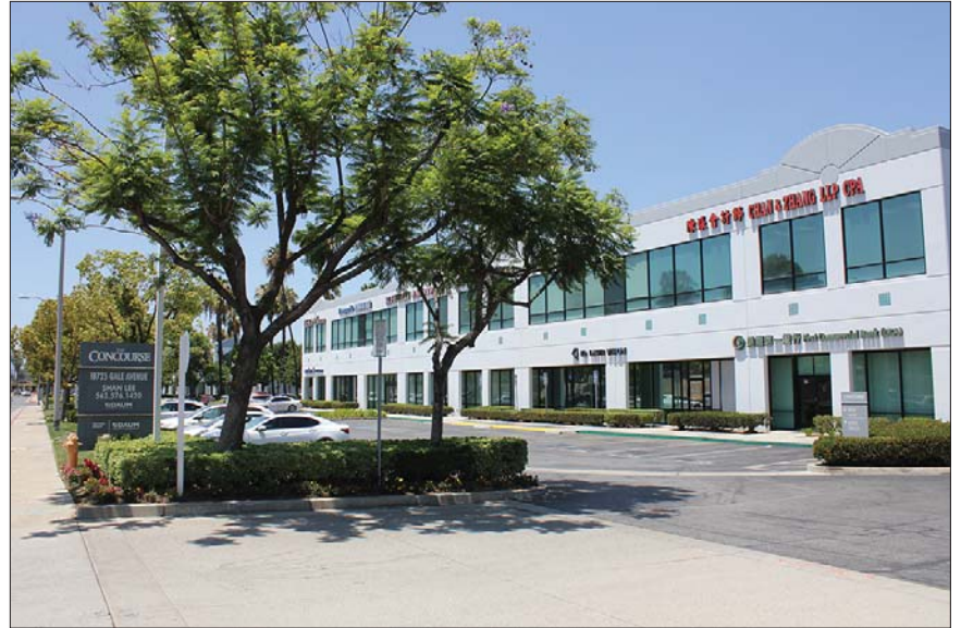
Photograph 2: The Concourse Business Park, west of Project Site on Gale Avenue
